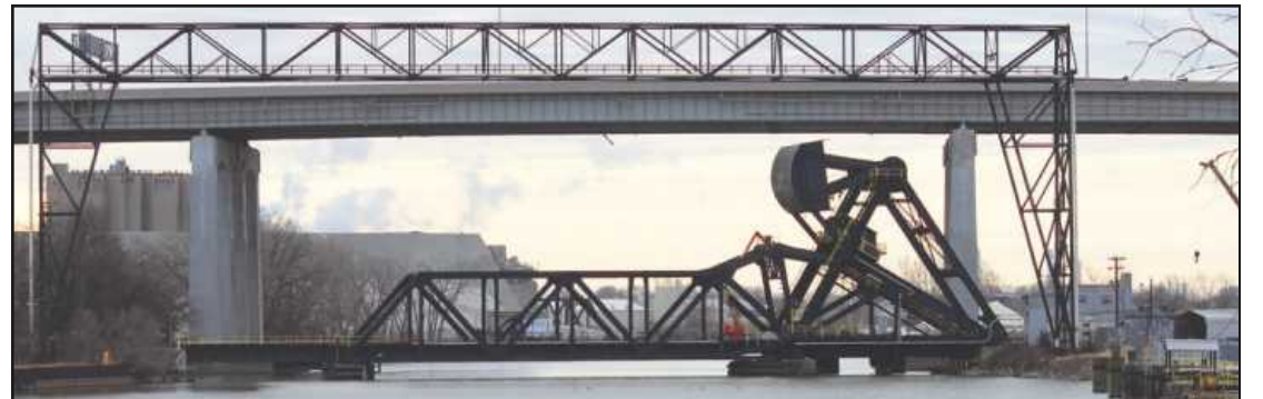
THE FIRST ABT/American Bridge bascule drawbridge design in Michigan, and the country, was built over the Rouge River in Detroit in 1922. Now framed by the I-75 bridge, iron workers renovated the still-active rail bridge for Norfolk-Southern last year.
